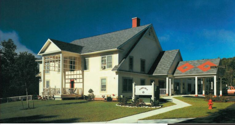
New construction of a 20,000sf, two level, wood frame building containing twenty-five apartment units. The work included asphalt shingle roof, wood/vinyl siding, standard interior finishes, elevator, hydronic heating system, 600 amp electric service, new paved roads & parking, and landscaping.
