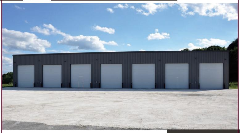
This project consisted of the new construction of a 12,000 sf, 7-bay metal preengineered building for the re-condonditioning services for a car dealership. Naylor & Breen worked with the aarchitect, NBF and Essex Steel on the building design and engineering.
