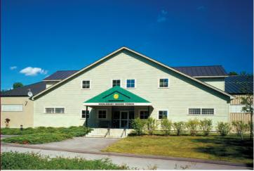
This project consisted of a pre-engineered steel building housing three tennis courts with a combination two story attached support building which houses the lobby, tennis shop, locker rooms and gathering facilities. Included was a "state -of -the-art" playing surface on the courts.
