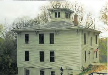
This project consisted of the complete renovation of a historic marble residence and separate wood frame carriage barn creating fourteen units of elderly housing; work included shoring, bracing, and lifting of carriage barn to construct a new
