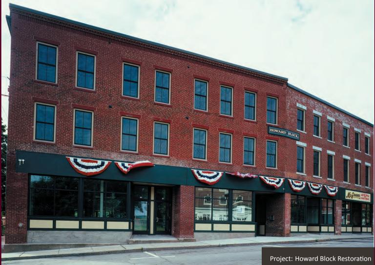
This project consisted of the restoration of a three story building known as the Howard Block, located in downtown Bellows Falls, Vermont. The work included renovation of the building's interior and exterior to provide 13 apartments, 6 shops, a new public foyer, a new elevator, and included new heating, plumbing, sprinklers,
