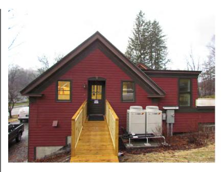
Vermont Land Trust—A historic rehabilitation paired with a new addition to provide adequate office space for staff. The existing historic structure was overhauled with a new HVAC system, lighting, attic insulation, and all new ceiling, wall, and floor finishes.
