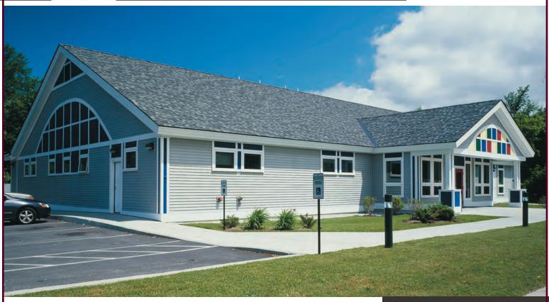
This project consists of a wood-frame, single story, slab on grade structure designed to provide exam rooms and doctors' offices.
