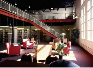
This was an extensive rehab, the bulk of which involved converting a college size gymnasium into a two level library. The new mezzanine level of the library was constructed of structural steel with a metal deck which was painted and exposed as finish.
