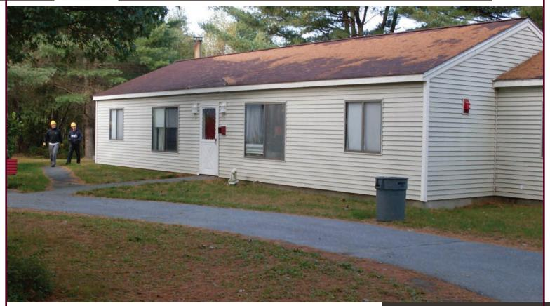
Located in White River Junction, VT, Graystone Housing Project consisted of extensive energy efficiency improvements. Naylor & Breen replaced all windows, doors, roofing, insulation and vinyl siding.
